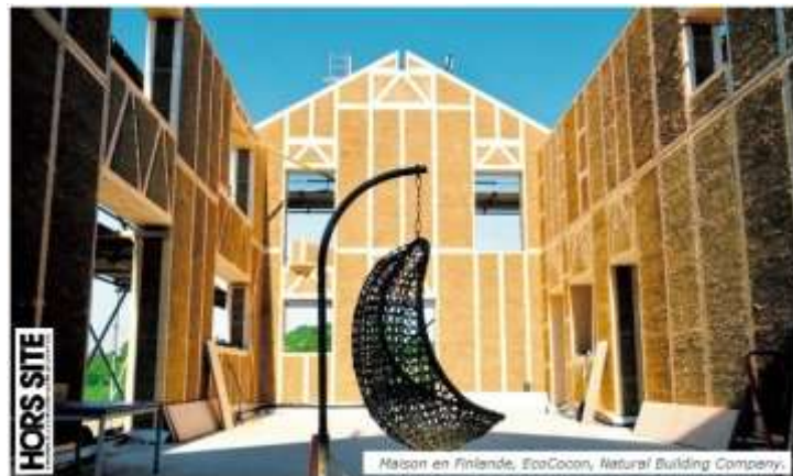
Maison en Finlande, EcoCocon, Natural Building Company.
